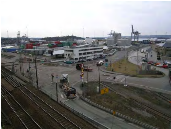
Figure 10: View from above of the roundabout at Sjursøya junction.
