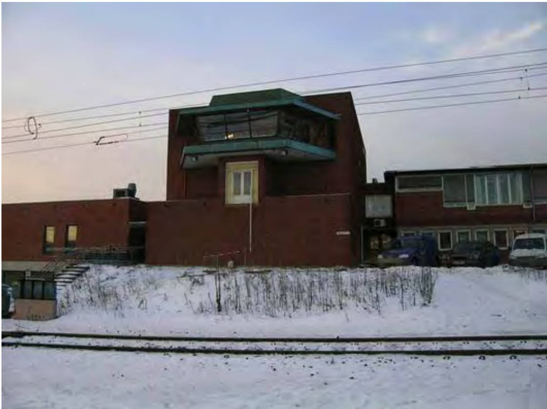
Figure 9: Alnabru Central Control Tower.
