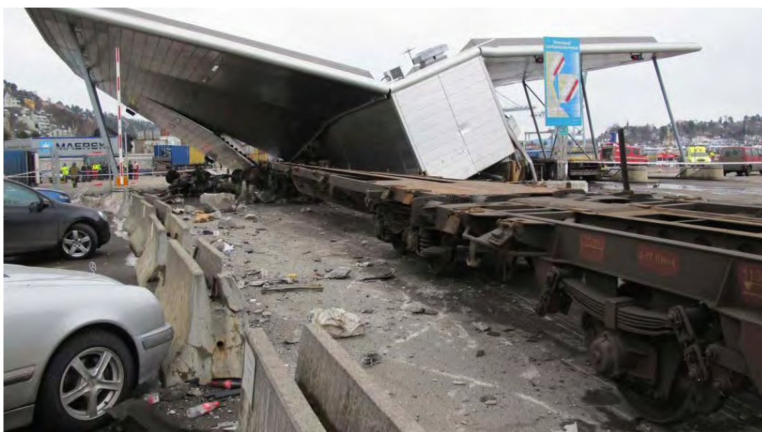
Figure 3: Photo of container terminal at Bekkelagskaia.
