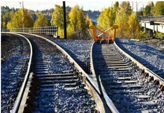
Figure 25: New run-off points at Alnabru South. (Photo: the NNRA)
