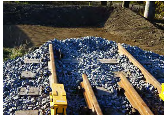
Figure 26: Sand drag after sliding buffer stops. (Photo: the NNRA)
