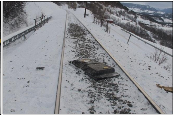
Figure 6: Strail panel at Hjelle level crossing finding G
