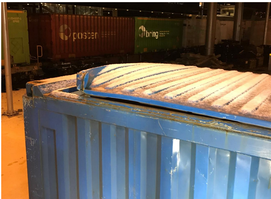
Figure 2-5: Photograph of the roof of the container which caused the damage to snow shelter structure at Stokkalia. Photograph: courtesy of Hans Bjørnseth.
