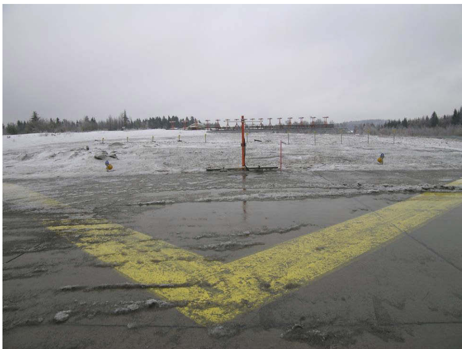
Figur 2: Reparert Localizer Monitoring antenne.
