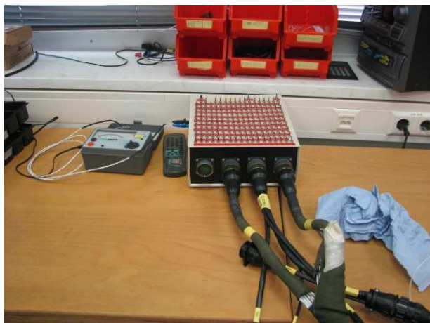
Picture 8 Isolation test set-up
