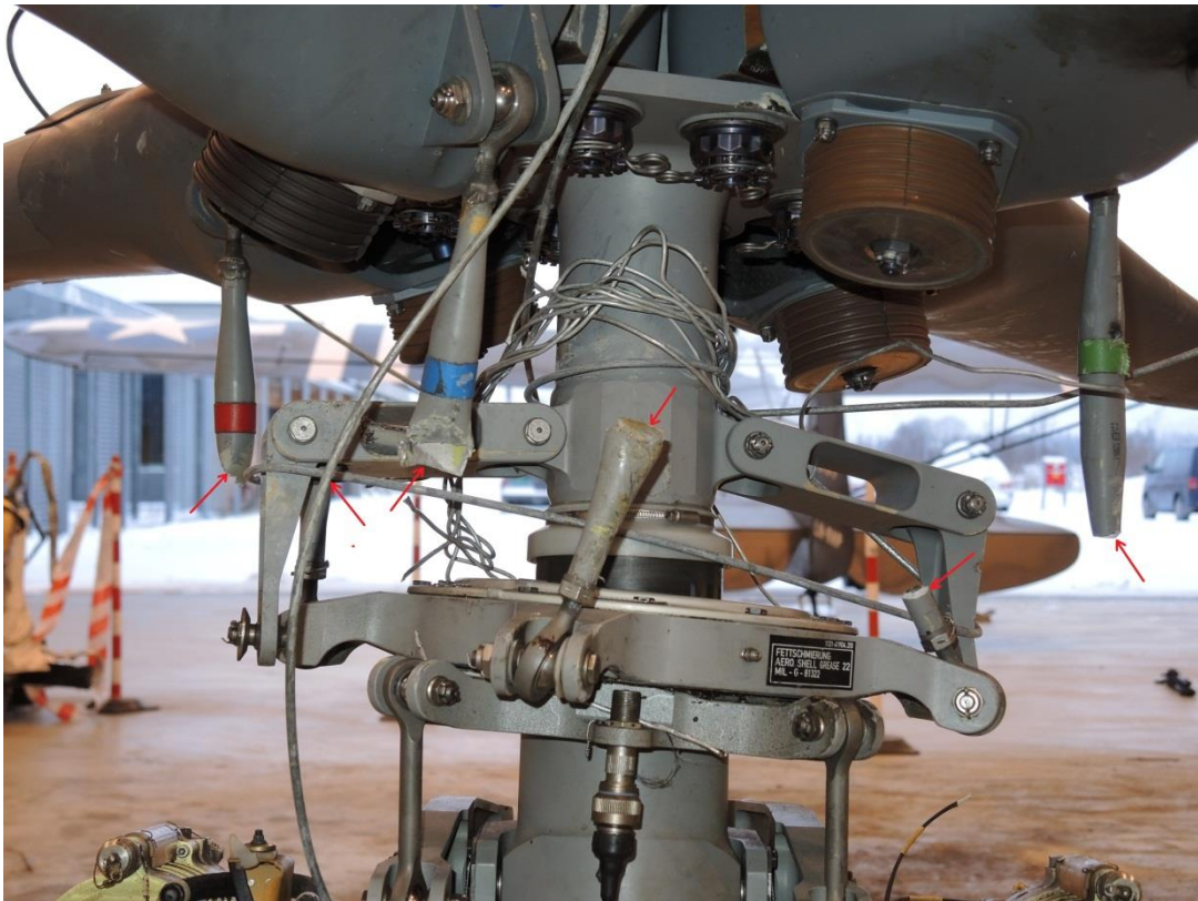
Figure 17: Rotor head, rotor mast, pitch mechanism and parts of the power line. Cut pitch links are marked with red arrows. Photo: AIBN
