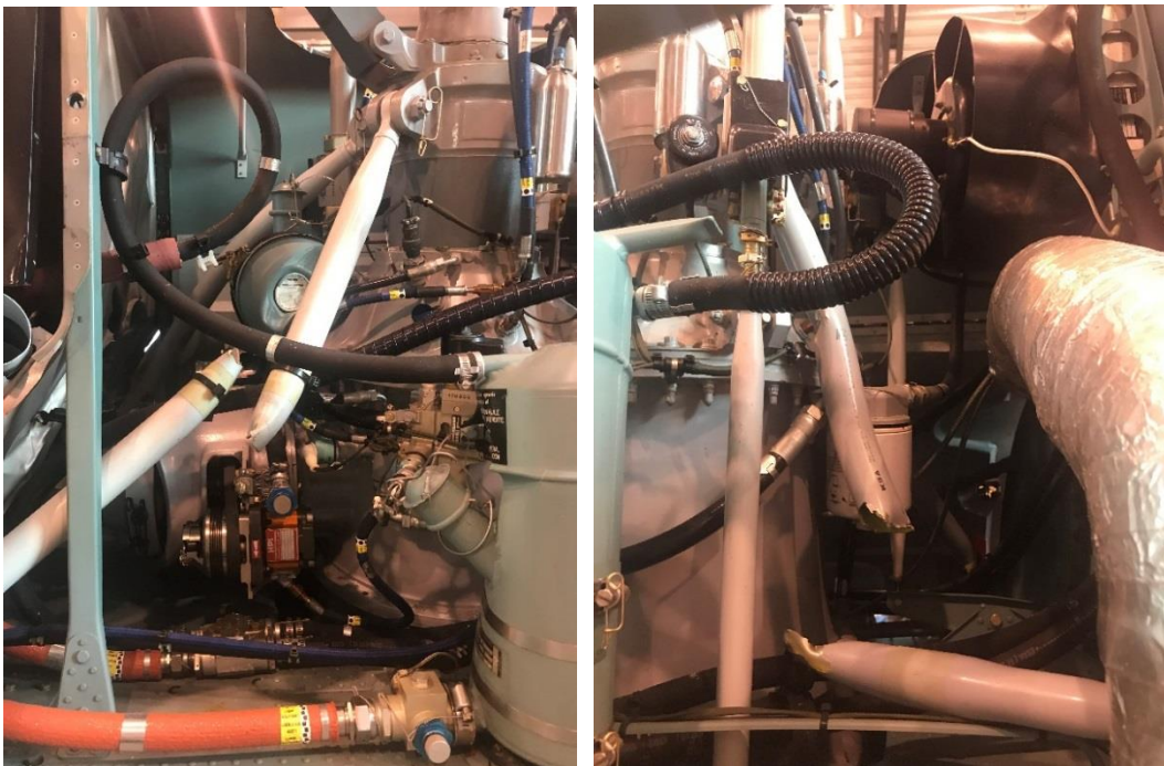
Figure 8: Forward and aft right hand MGB suspension bars. Photo: AIBN
