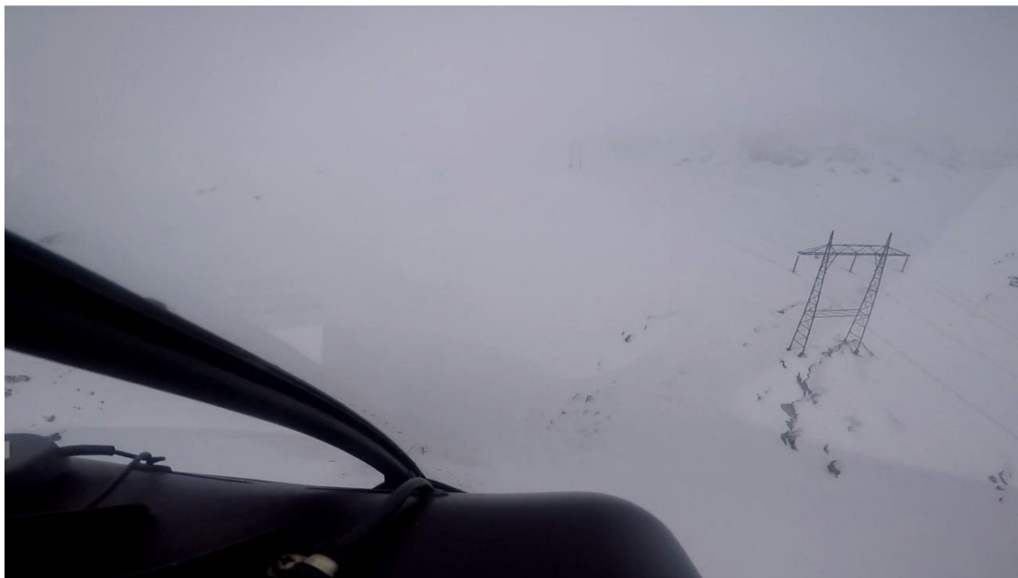
Figure 5: The LN-ORH flying along the power line at a low altitude. One pylon to the right and the next pylon are barely visible near the middle of the photo. Source: Video from the helicopter
