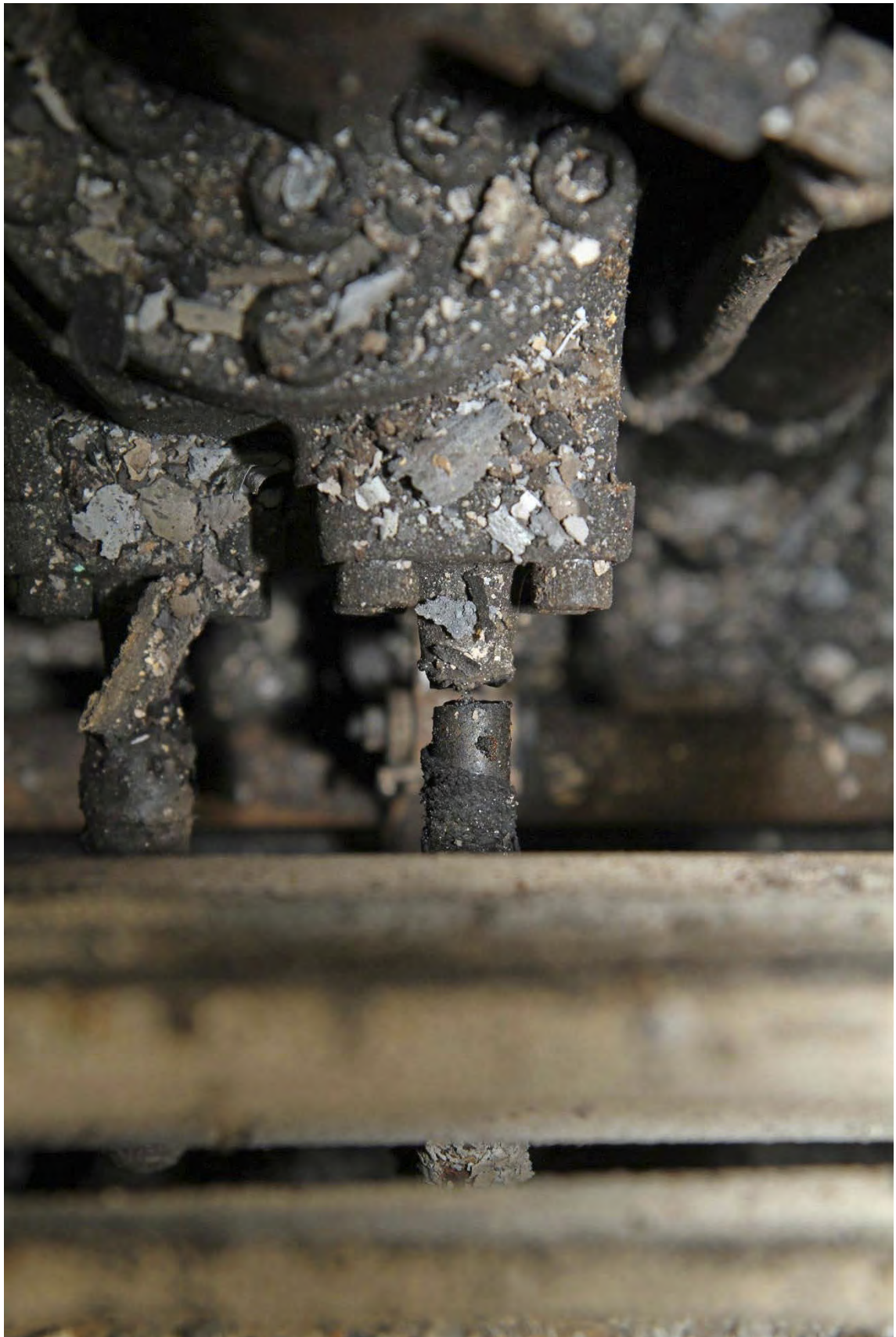
Figure 16: The breakage in the fuel return pipe (see ref. 4) in Figure 15) where it was attached to pump no 5, viewed from above. Photo: The police.
