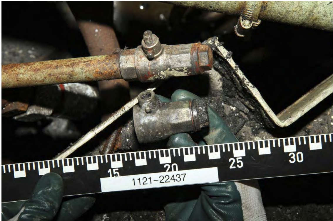
Figure 20: The drainage valve from the starboard main engine held next to the drainage pipe with valve on the port main engine. Photo: The police.
