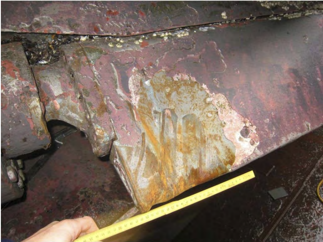
Figure 38: The photo shows the marks/damage sustained on the starboard stabiliser fin, at the end closest to the hull, after it penetrated the skin. Photo: DNV.
