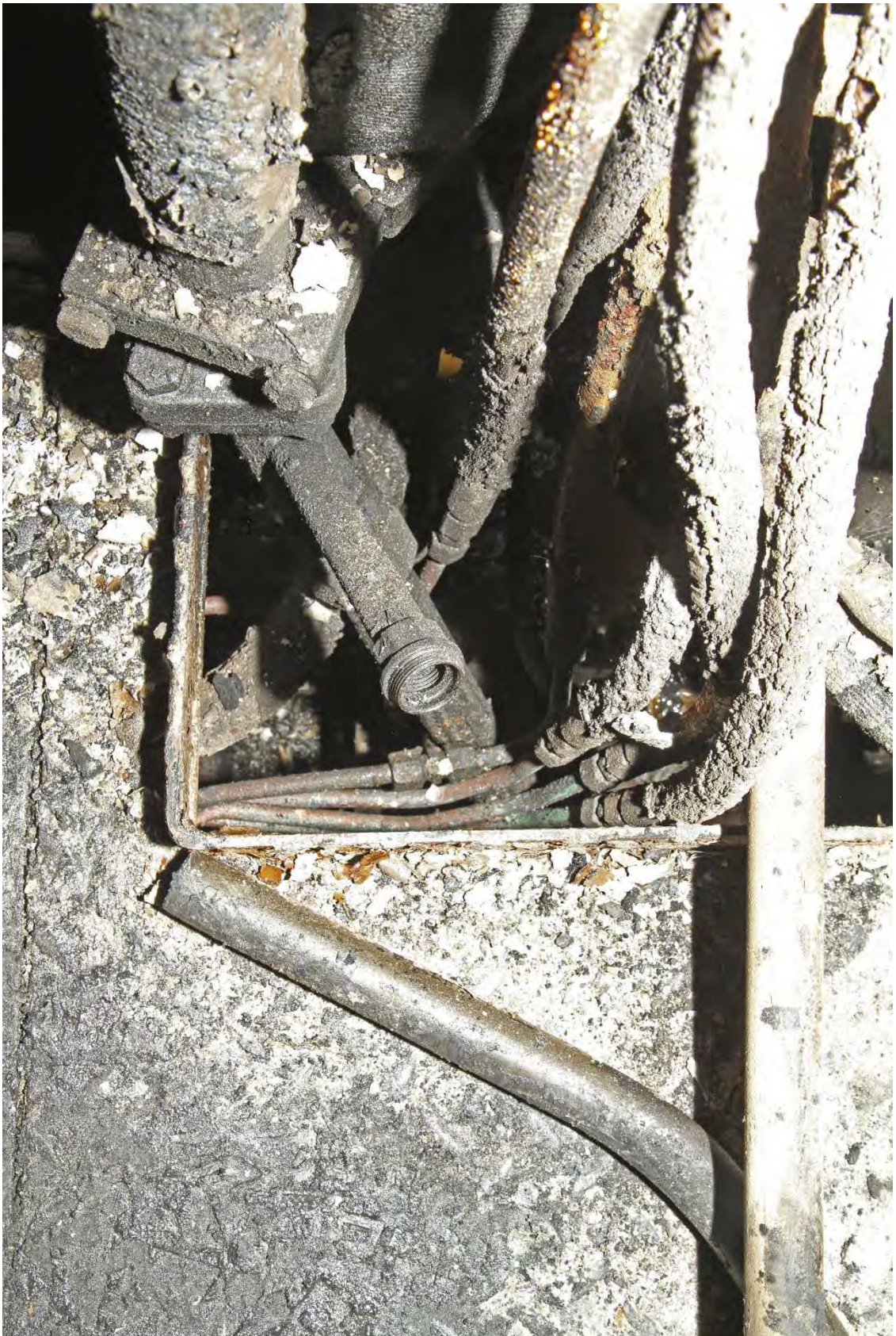
Figure 19: Drainage pipe on starboard main engine, without valve. Photo: The police.
