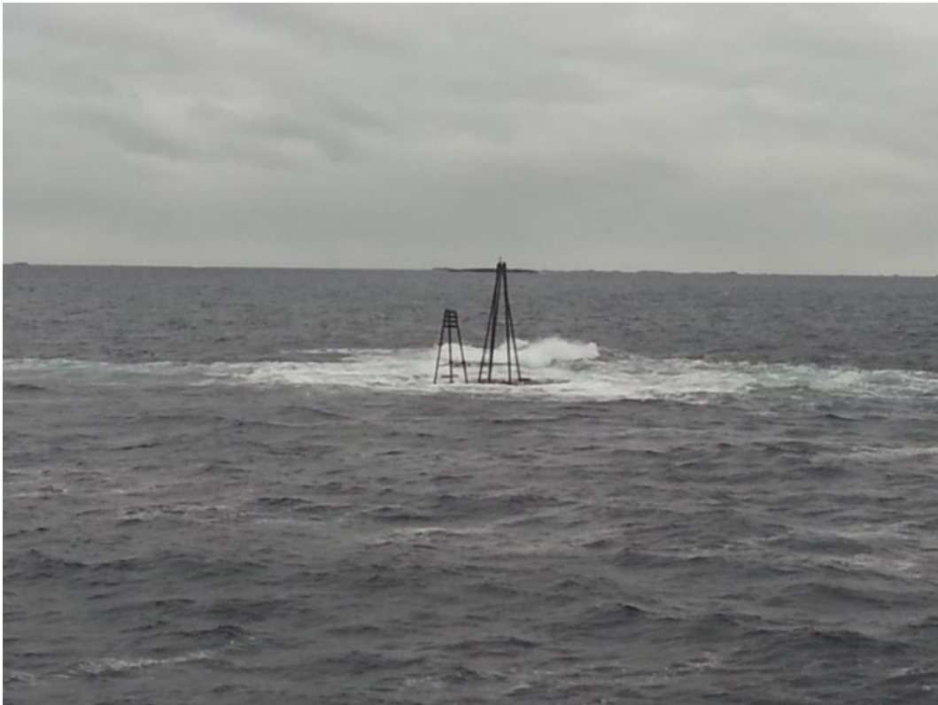
Figure 3: Brakan, November 2014, around high tide. A provisional navigational installation is in place to the right of the old beacon, as was also the case at the time of the accident. Photo: The Norwegian Coastal Administration (NCA)
