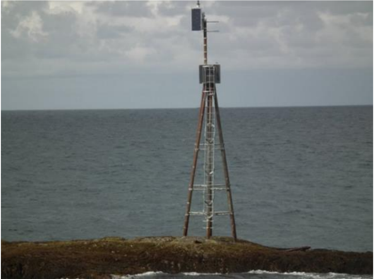
Figure 8: The beacon at Brakan was first lit on 15 July 2015. Photo: The Norwegian Coastal Administration (NCA)
