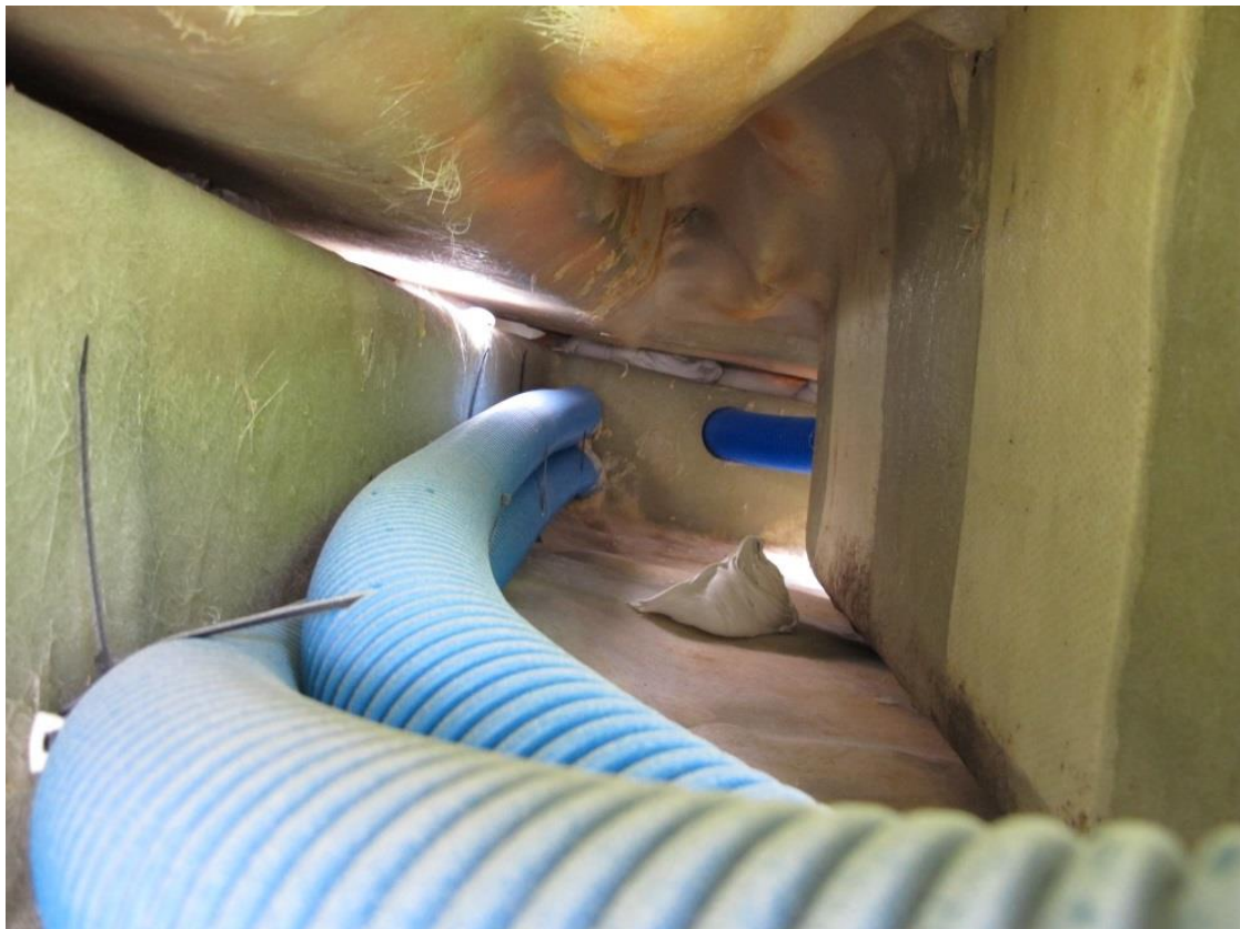
Figure 19: Volume (not filled with foam) below inner liner on the starboard side of the wheelhouse. Photo taken from the forward end, looking towards the stern. Photo: AIBN
