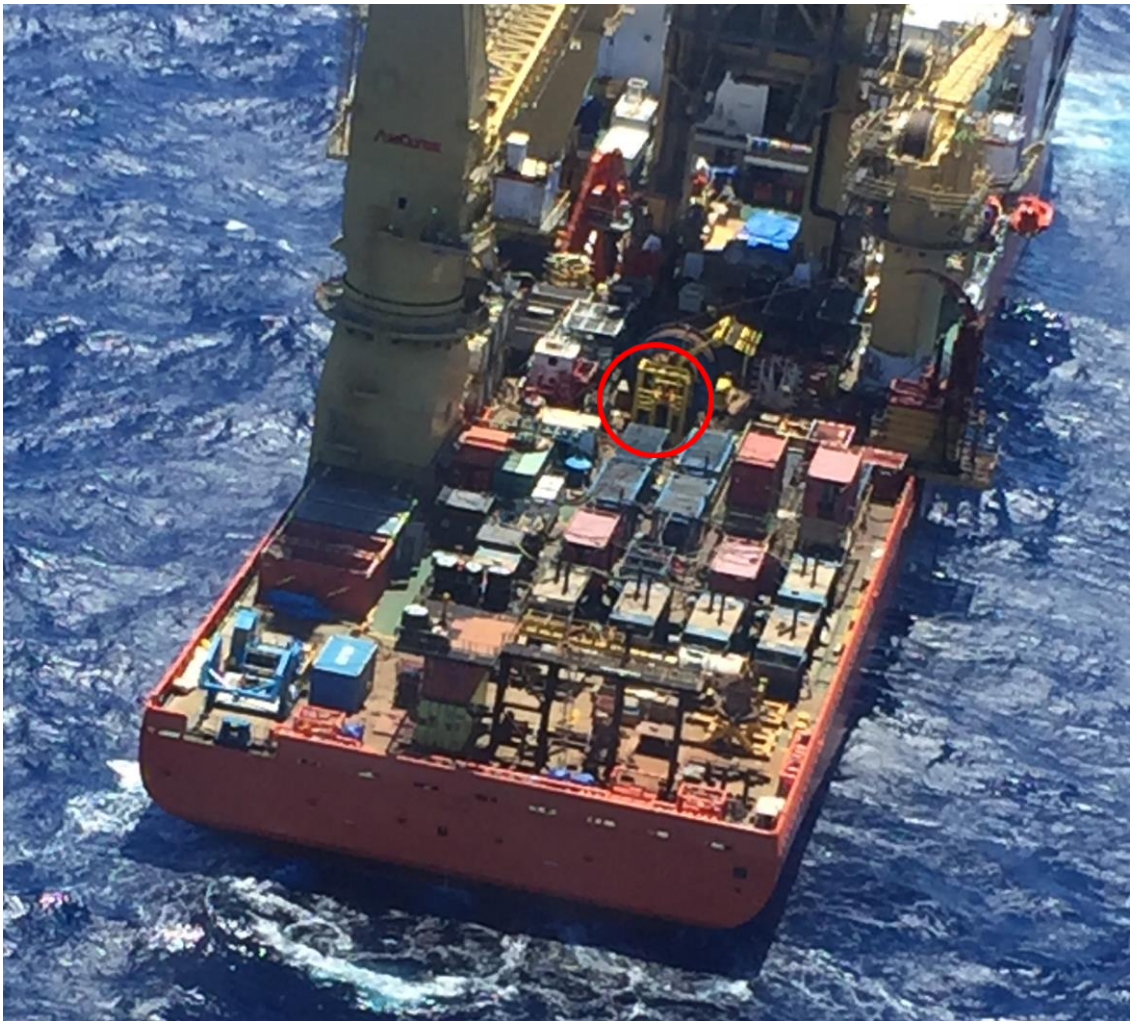
Figure 3: The system installed for use in the pre-commissioning assignment consisted of a number of components placed on the open aft deck of the CSV Normand Maximus. The accident site is marked with a red circle. Photo: The Brazilian Navy
