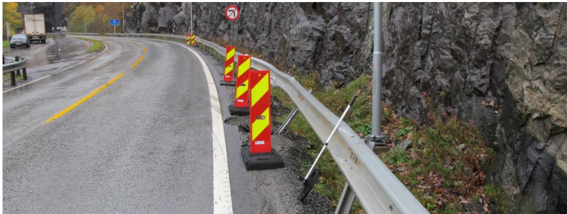
Figure 8: Damages to the crash barrier looking westwards. The closest barrier posts mark the final position of the westbound heavy goods vehicle. Approximately 30 m behind them in the photo, we find marks from the eastbound semi-trailer. The photo was taken the day after the accident. Photo: AIBN
