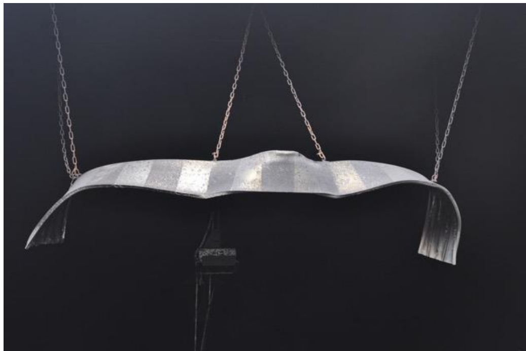
Figure 16: A photograph taken after the fire of the height limit sign at the Hamnen portal (source: NPRÅ).
