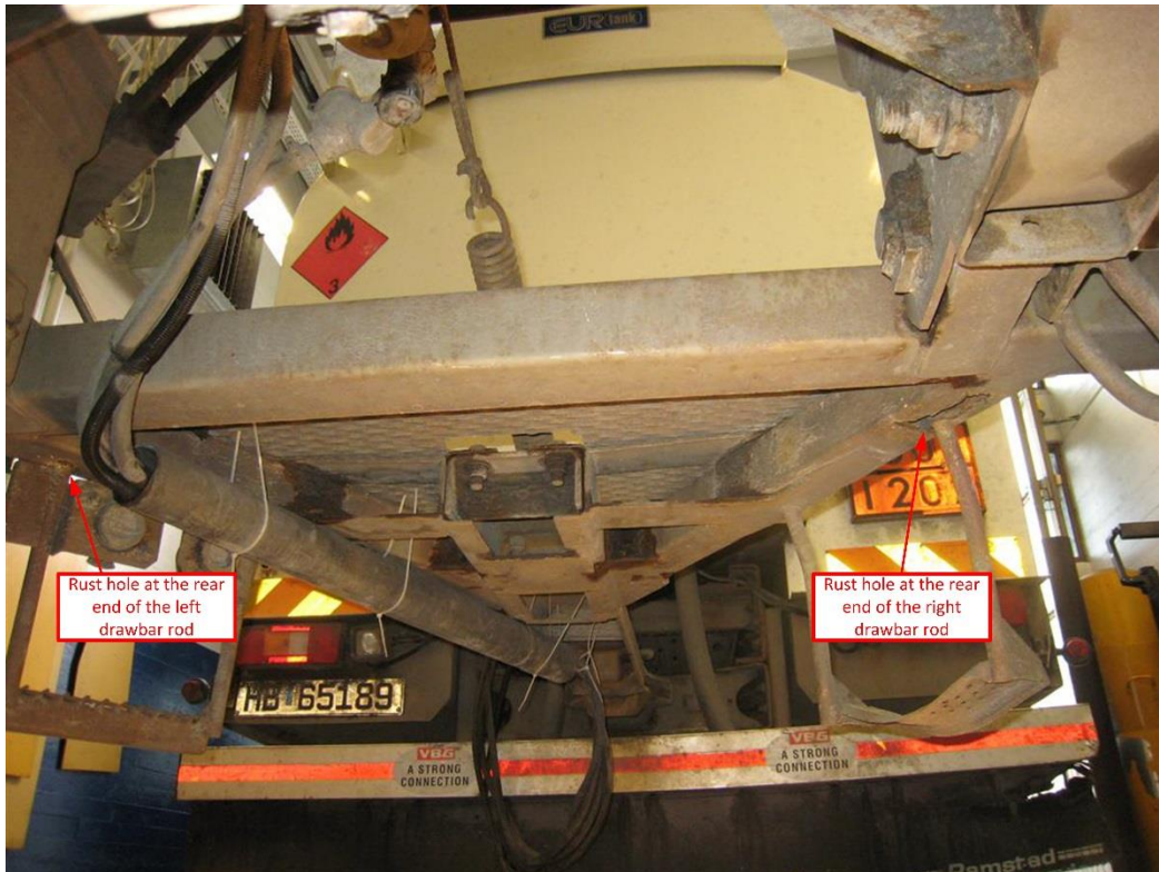
Figure 12: Rust damage to the drawbar found in the NPRA's inspection of the trailer in May 2011. Photo: NPRA
