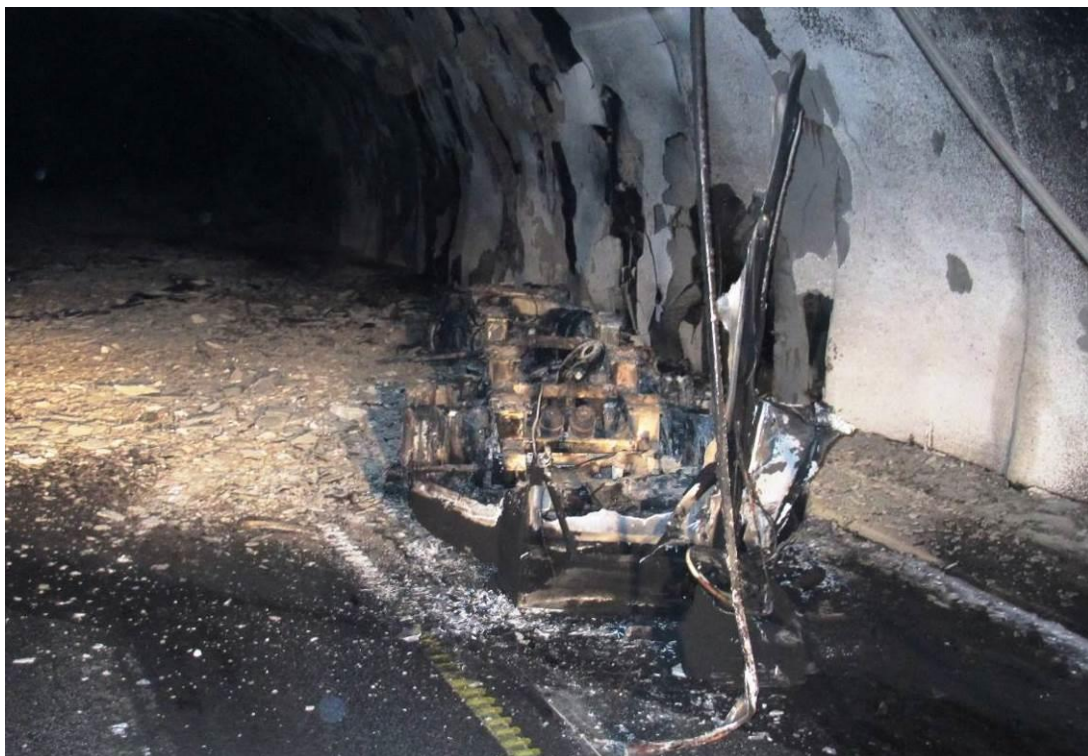
Figure 4: The remains of the tank trailer as left behind when it had broken loose from the truck. Photo: AIBN
