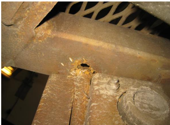
Figure 13: Rust damage in left drawbar rod. Photo: NPRA
