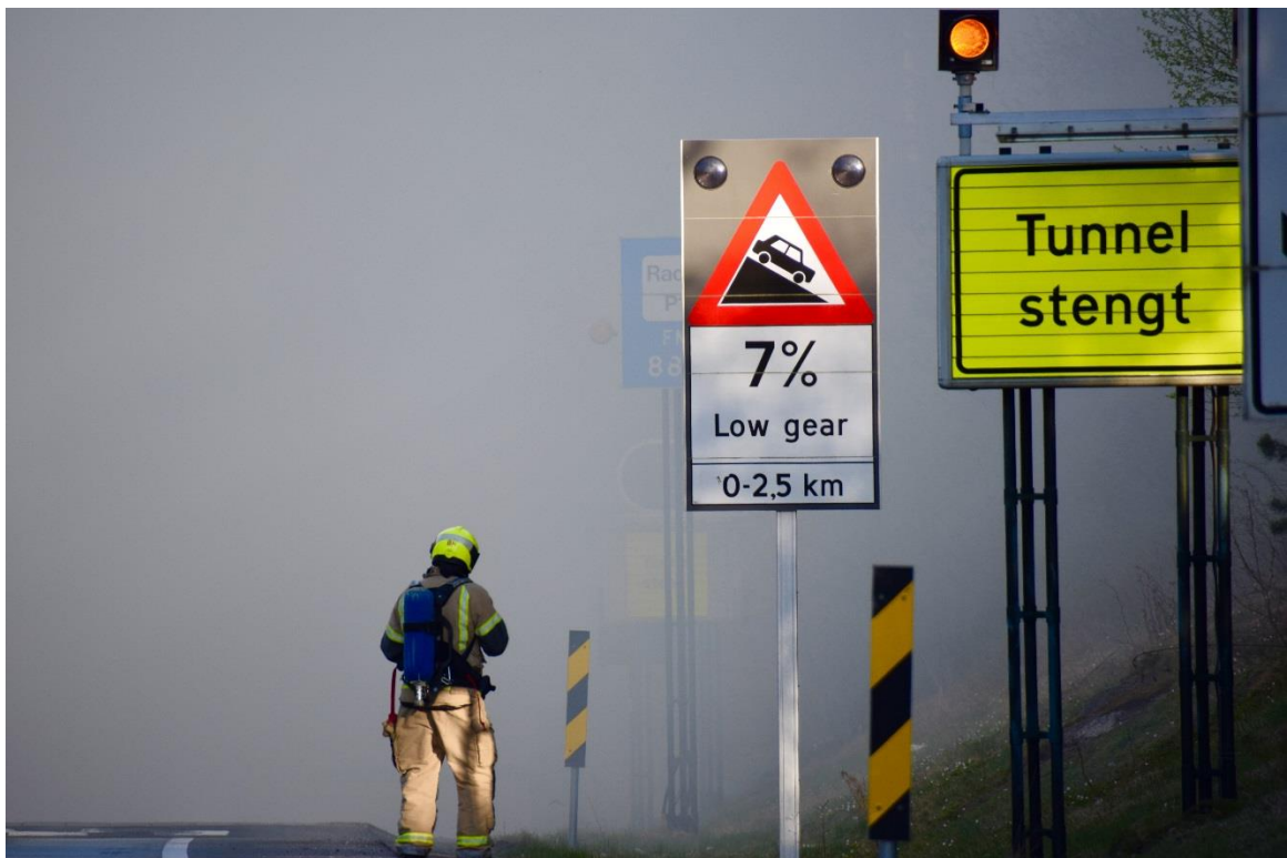
Figure 12: Smoke from the Oslofjord tunnel during the fire on 5 May 2017. Photo: Edgar Dehli
