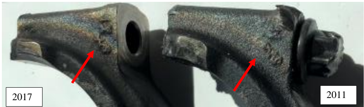
Figure 41: Bearing cap fastening from 2017 (left) and 2011 (right) with discoloration caused by heat. Photo: AIBN
