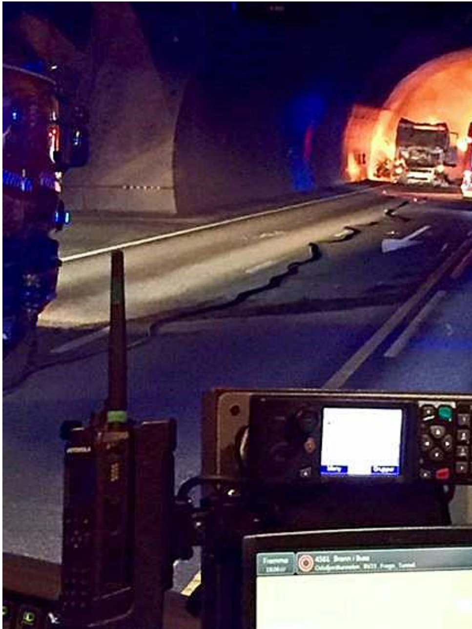
Figure 8: View from the cabin of FBV's purpose-built tanker used during the extinguishing efforts in the Oslofjord tunnel on 5 May 2017. Photo: Follo fire service IKS
