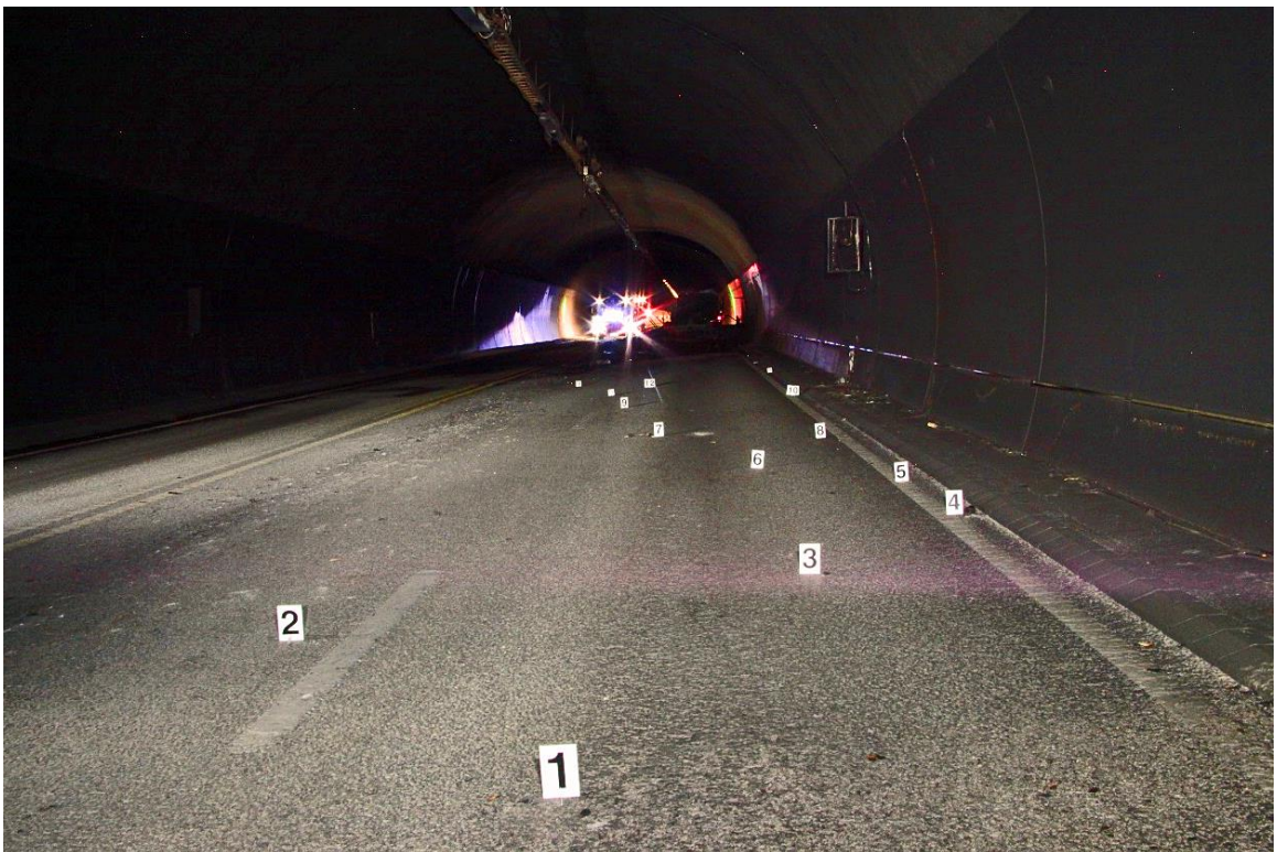
Figure 16: Engine parts from the heavy goods vehicle scattered on the road. Photo: The police
