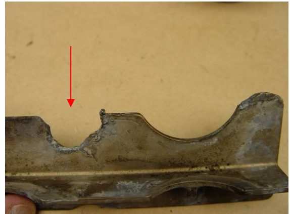
Figure 12: The bracket holding the oil transfer tubes. The arrow points at the fracture.
