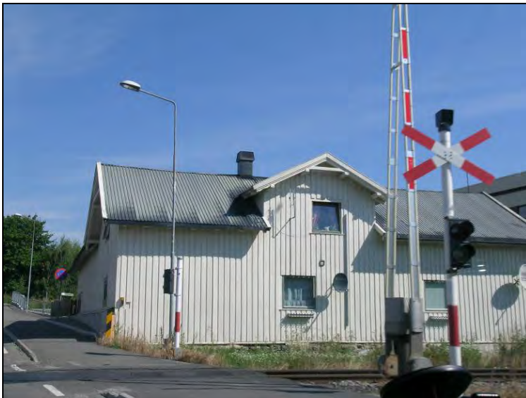
Figure 48: Extra red light signal at the top of a St Andrew's cross.
