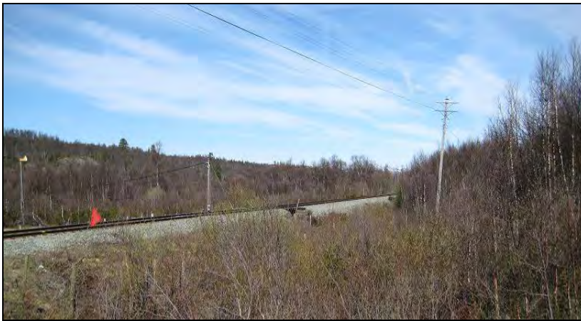
Figure 45: Good sight lines at Nesvoll LC on the Røros line
