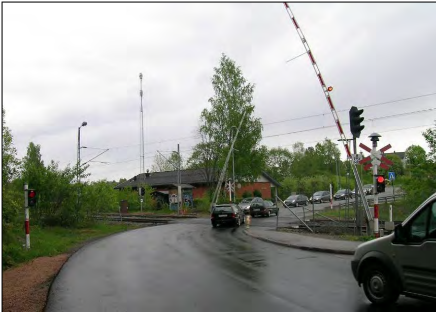
Figure 57: Example of poor traffic behaviour - two cars have managed to cross the level crossing before the light changes to white and the barriers have been fully raised
