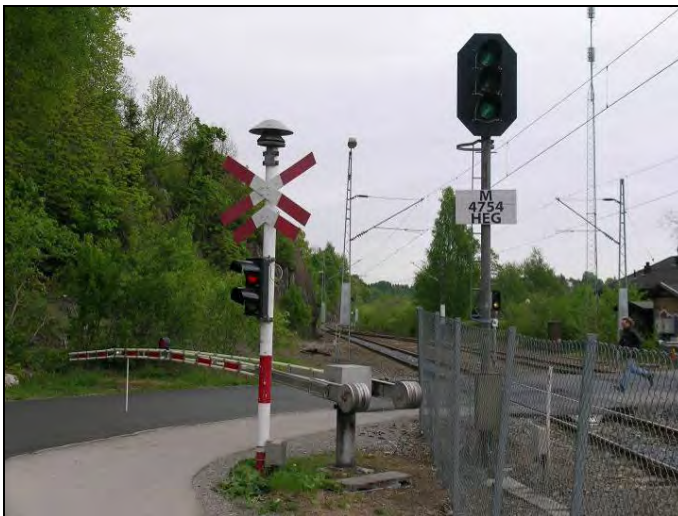
Figure 51: Would a stop line here have helped motorists to ascertain where the barrier comes down?
