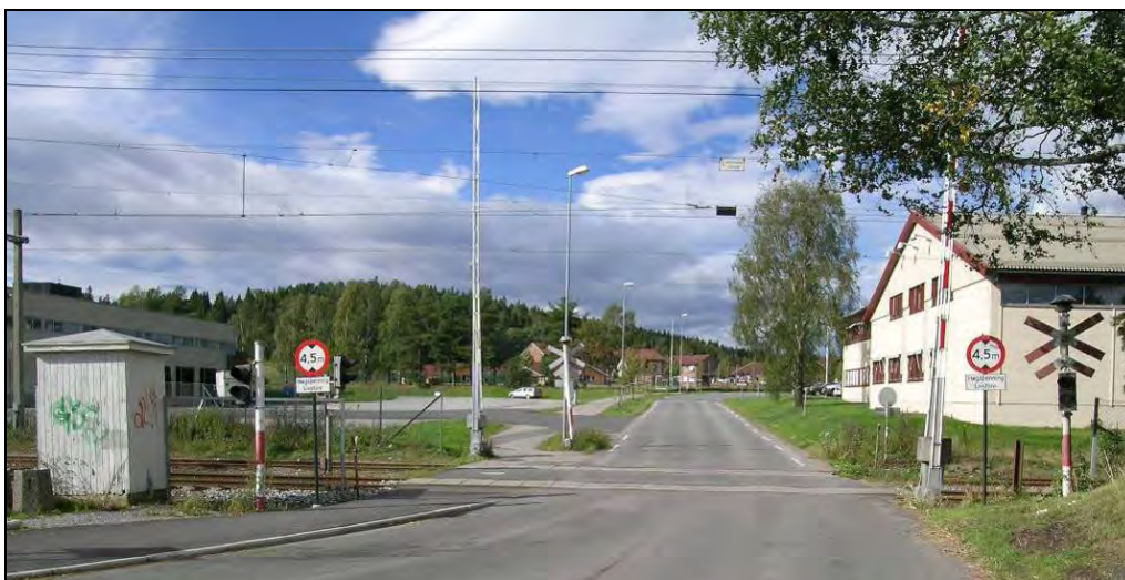
Figure 6: Example of a full barrier and well-marked road safety system (Spydeberg).
