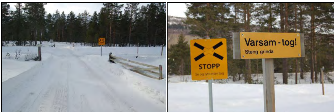
Figure 10: Example of gates and signs (a private level crossing on the Rauma line).
