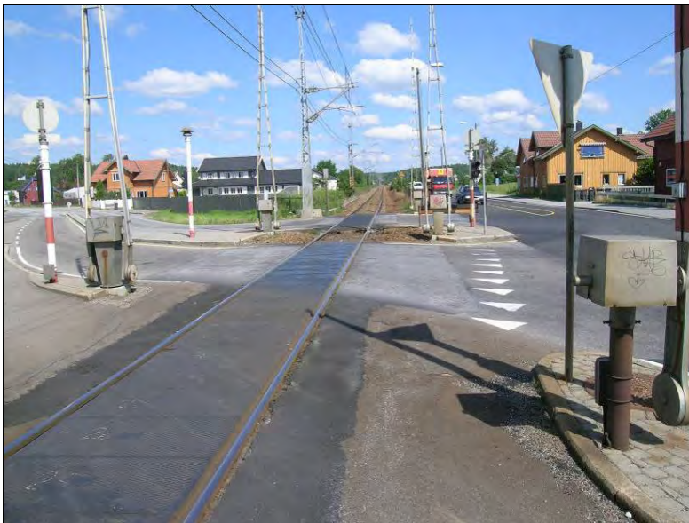
Figure 52: The give way line can mislead motorists into stopping too close to the track.
