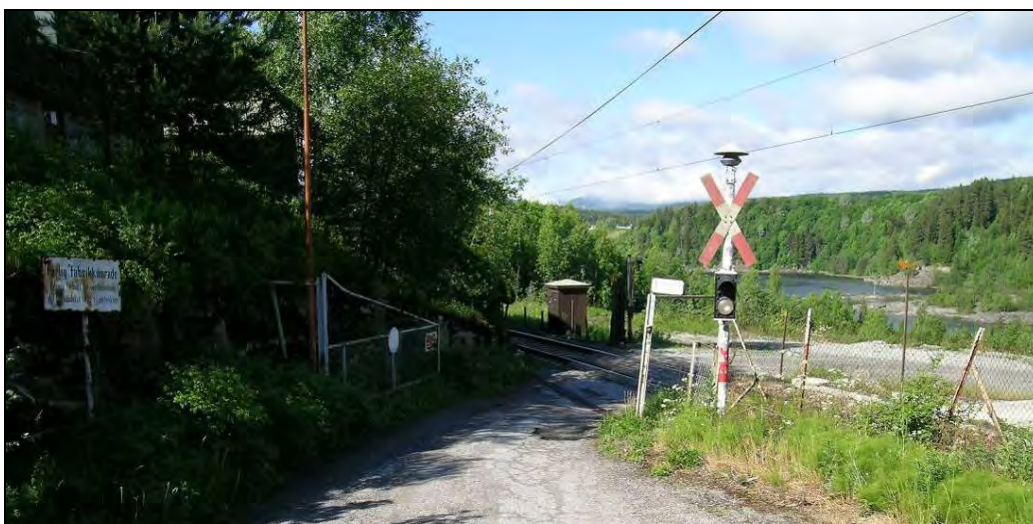
Figure 8: Example of sound and light signal (Embretsfoss LC before a full barrier system was installed).
