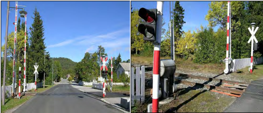
Figure 61: Barriers on the same side of the level crossing (Os LC).
