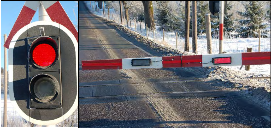
Figure 47: Shades highlighting the signal and alternating warning lights on the barrier.
