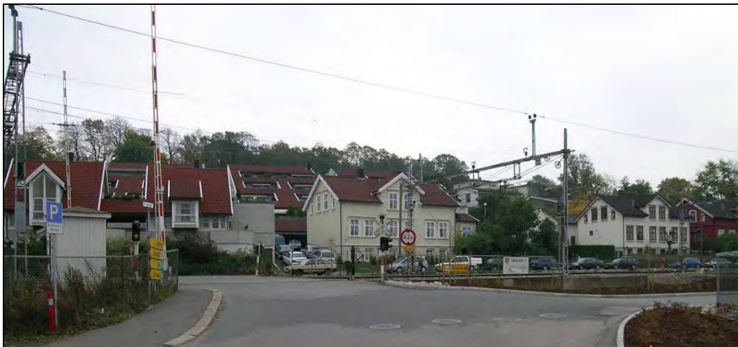
Figure 62: Barriers on the same side of the level crossing (Moss South LC).
