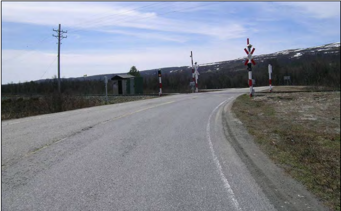
Figure 42: Inspection of Harborg LC on the Røros line.
