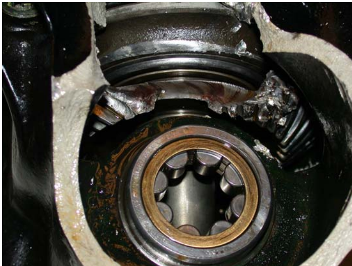
Figure 2 Photograph of fractured gear as observed in input side of the gearbox ref. Figure 1.
